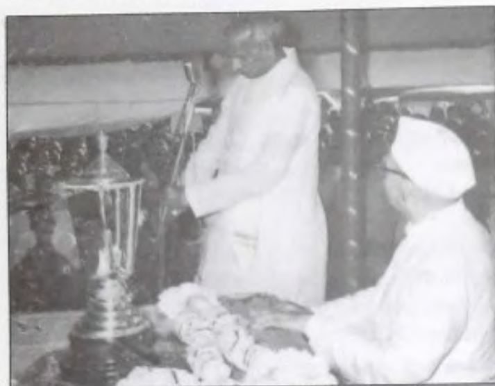
Hon'ble Minister for Defence Shri.V.K. Krishna Menon addressing the gathering on the occasion of the foundation laying ceremony of Sainik School Kazhakoottam on 5th Feb. 1962 in the presence of Shri. Pattom Thanu Pillai, Chief Minister of Kerala.
